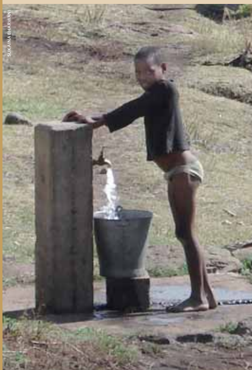
Despite agreements that services such as running water would be provided when the Mohale dam was built, they are often faulty or poorly maintained.
